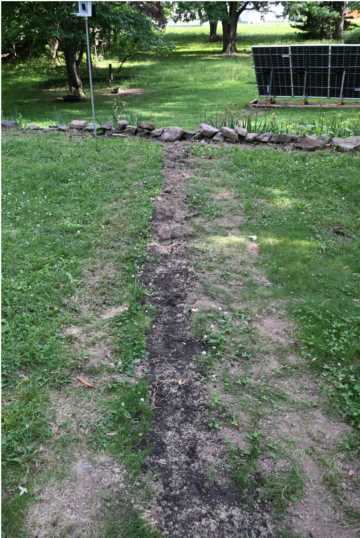
This photo shows the trench run (about 70 feet) back to the house. It was at two heights transcending a three foot stonewall midway.
