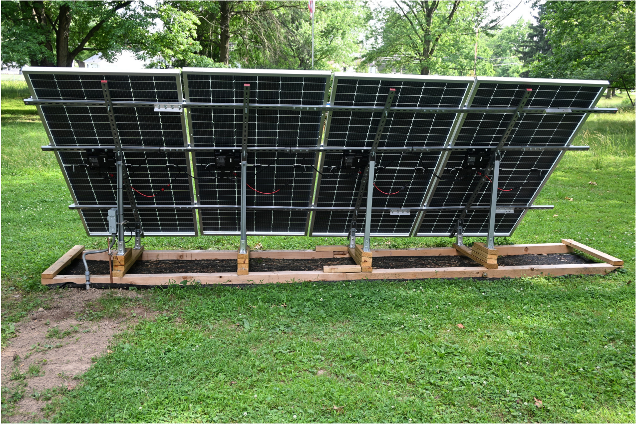
A view of the rear. Feed trench to the left.
