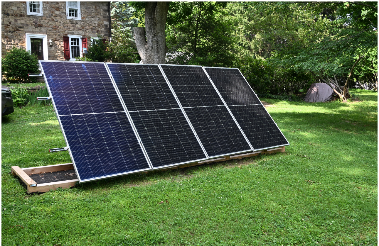
Two views with all four panels installed.
